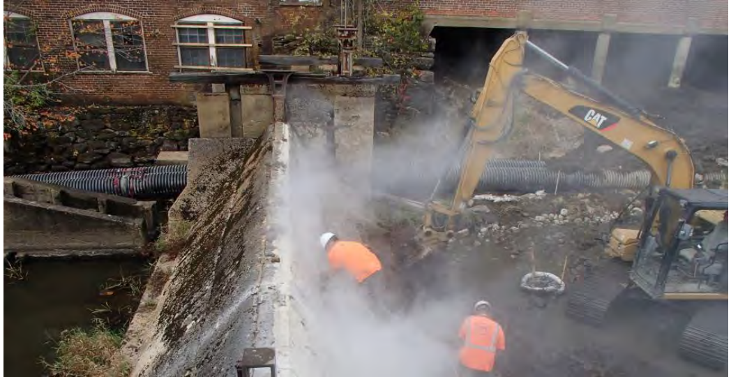
Cotton Gin Mill Dam Removal, East Bridgewater
